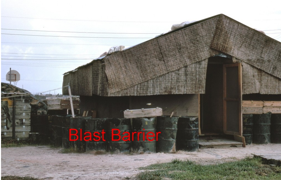
In this picture you can see the blast barrier of my hooch
